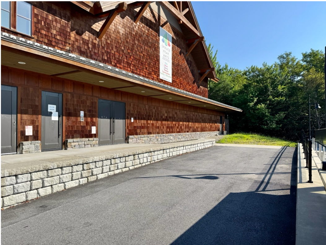
On Driveway showing Stage and Loading Doors
