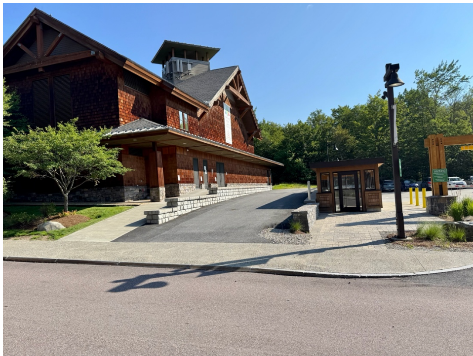
Entrance to Driveway on South side of SPA
