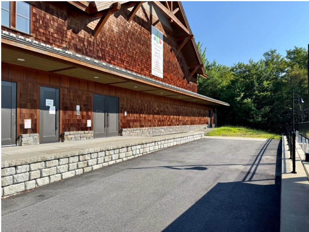
On Driveway showing Stage and Loading Doors
