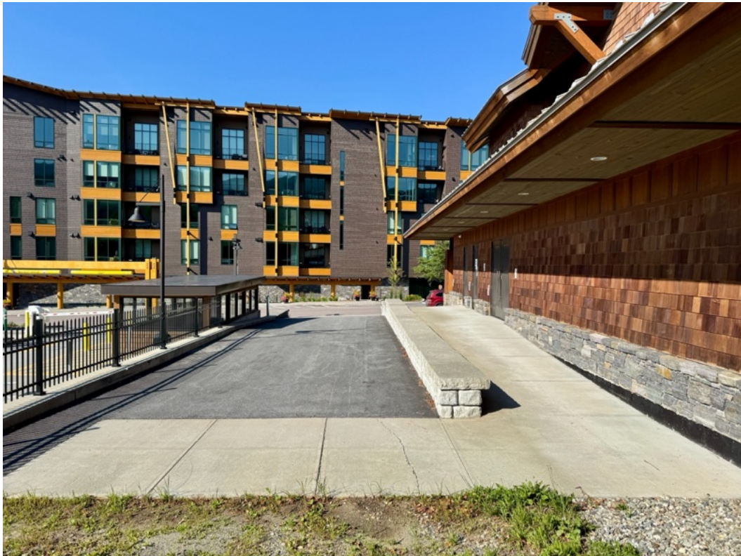
On Driveway looking back at Hourglass Dr with Loading Ramp on Right
